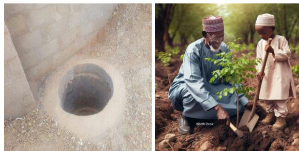
Figure 2. Picture of a local well under construction by the Waqf institutions and Tree Planting Project
